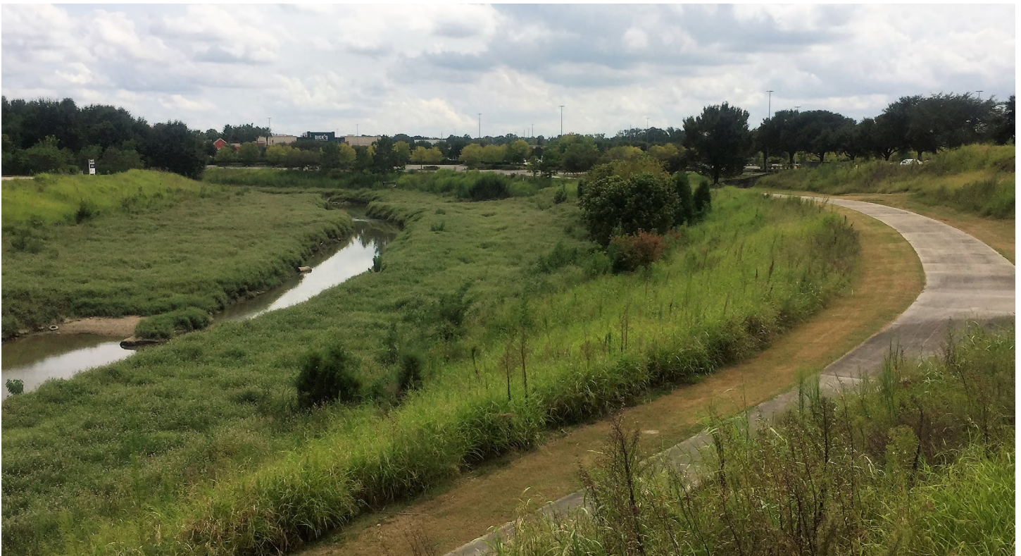
Bluebonnet storm water detention, Baton Rouge
